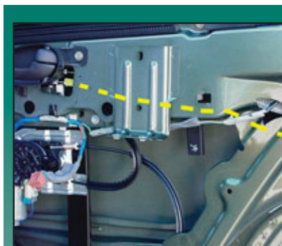
2. The dotted line indicates the position of the horizontal control linkage rod.
